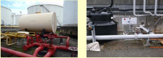
Storage material, pipework, valve seats, etc
